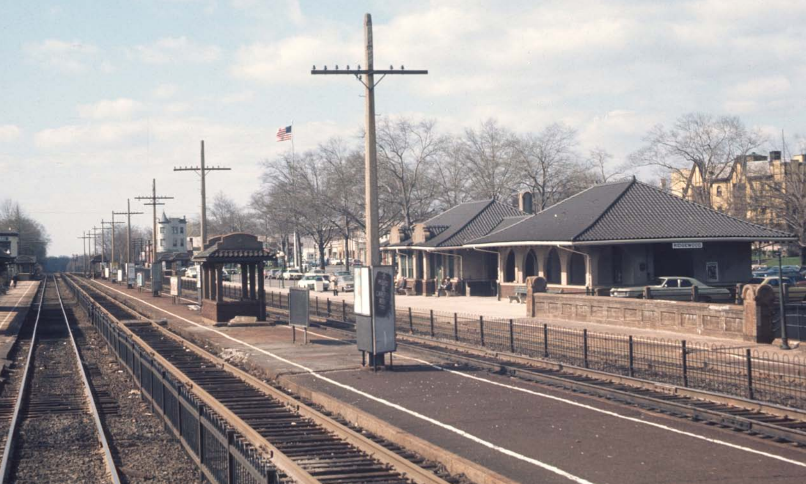
Above. (Mike Pagano collection Circa 1974) Ridgewood Station (MP 20.9) sports the southwest stucco style architecture on an elevated right of way. Originally, four tracks ran from Ridgewood Junction to Waldwick and beyond. Now there are three tracks in this location but the station is still a major station stop and utilizes the original pedestrian entrance tunnels to reach all the platforms.
