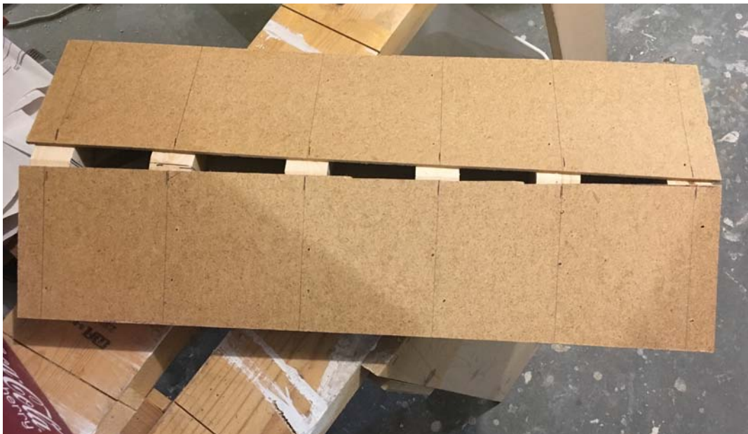
Left. The roof was cut from scrap 1/8" Masonite. I realized my pieces were not straight and did not meet at the peak. I thought ahead and realized that the bottom had to be square but the clerestory could hide the gap at the peak.
