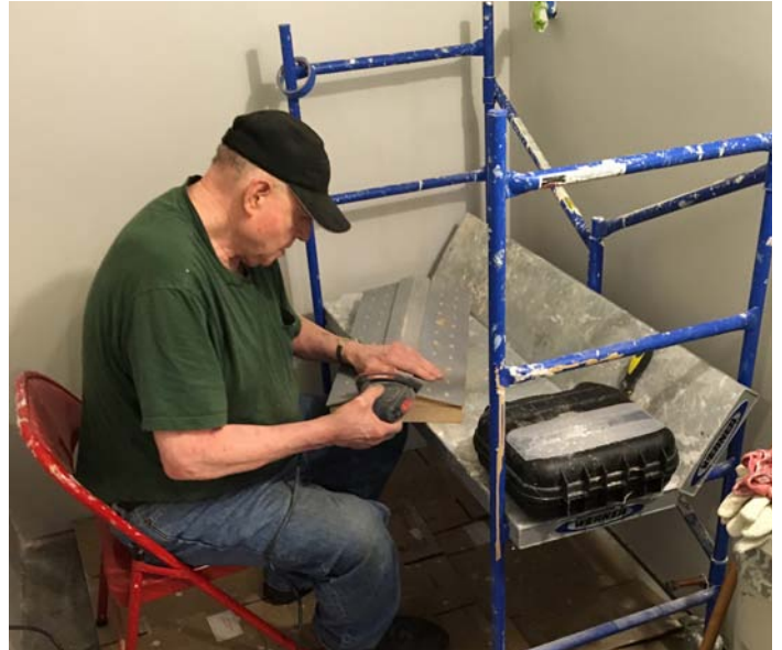
Above. He removed my vents and sanded the roof with an electric pad sander.
