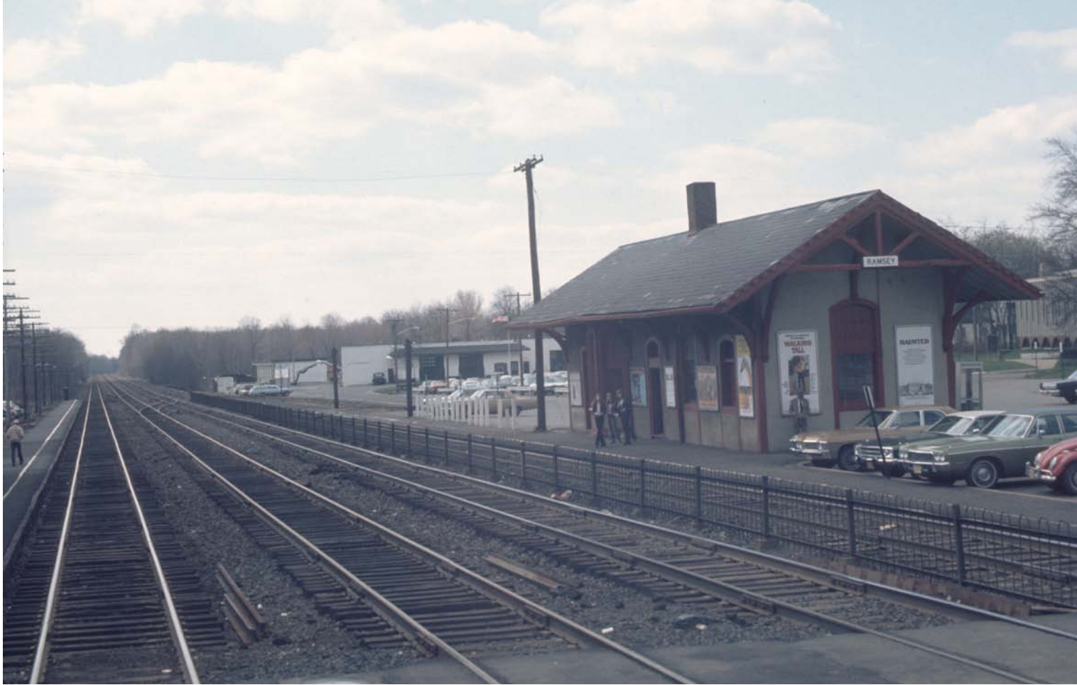
Above. (Mike Pagano collection Circa 1974) The Ramsey Station (MP 26.6) might look familiar in an Atlas Railroad catalog. It's a typical Erie station design that was also used in Maywood, New Jersey.
