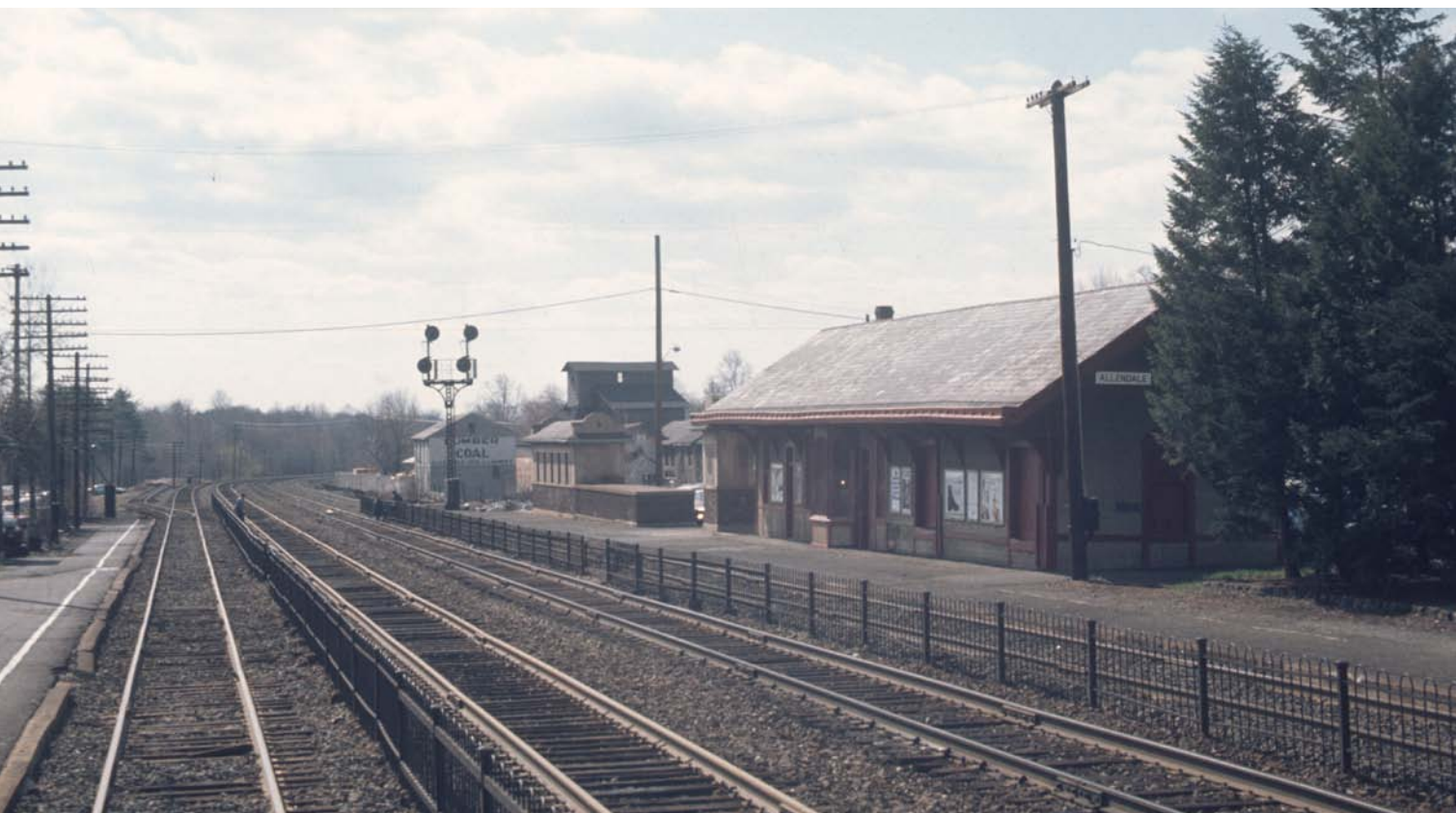
Above. (Mike Pagano collection Circa 1974) Allendale Station (MP24.7) was built in the late 1800s. By 1902 the structure was moved to the opposite side of the tracks as the right of way was expanded from two to four tracks during the Erie era.
