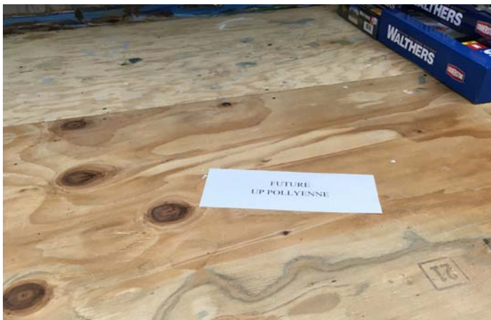
41 Above. On the other side of the barrier.
