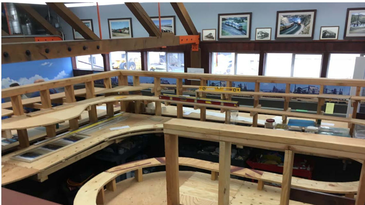
20 Above. Another view of the sub roadbed of the Southern Pacific mainline.
