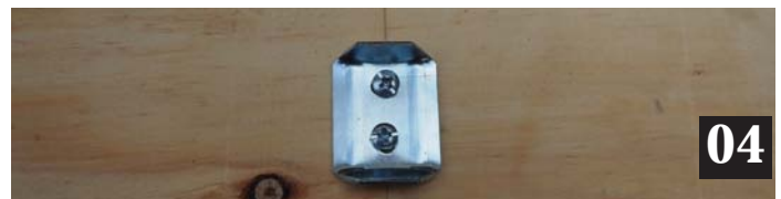
Step 04: On the center line at about 50mm in from the top drill and screw on the toilet roll retaining bracket.
