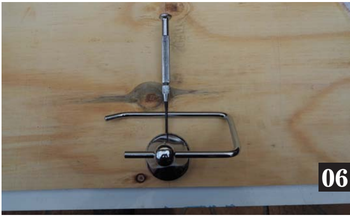
Step 06: Then tighten the attachment screw.
