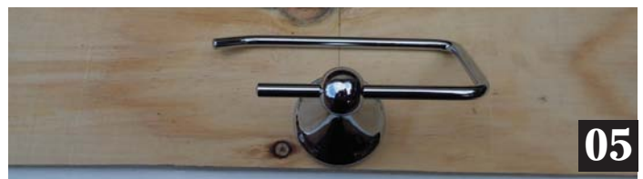
Step 05: Align and place the toilet roll holder over its retaining bracket.
