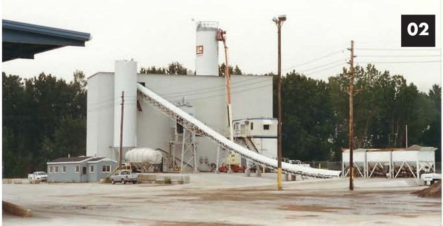
Image 02. Serv-All Concrete/Erie Sand and Gravel plant, Erie, PA. Ground bins feeding a single conveyor belt into enclosed plant structure. Two cement silos, ground mounted one in other photos for reference, Main silo has workers in man lift. Plant operator and truck dispatcher work from small elevated office.
