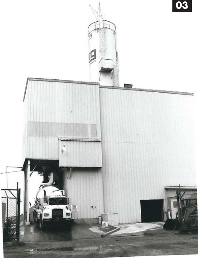
Image 03. The front of plant on a cold day. The truck is pulled under chute for loading by central mix barrel inside the plant. Make sure there is standing water around your model as there almost always is in the prototype.
