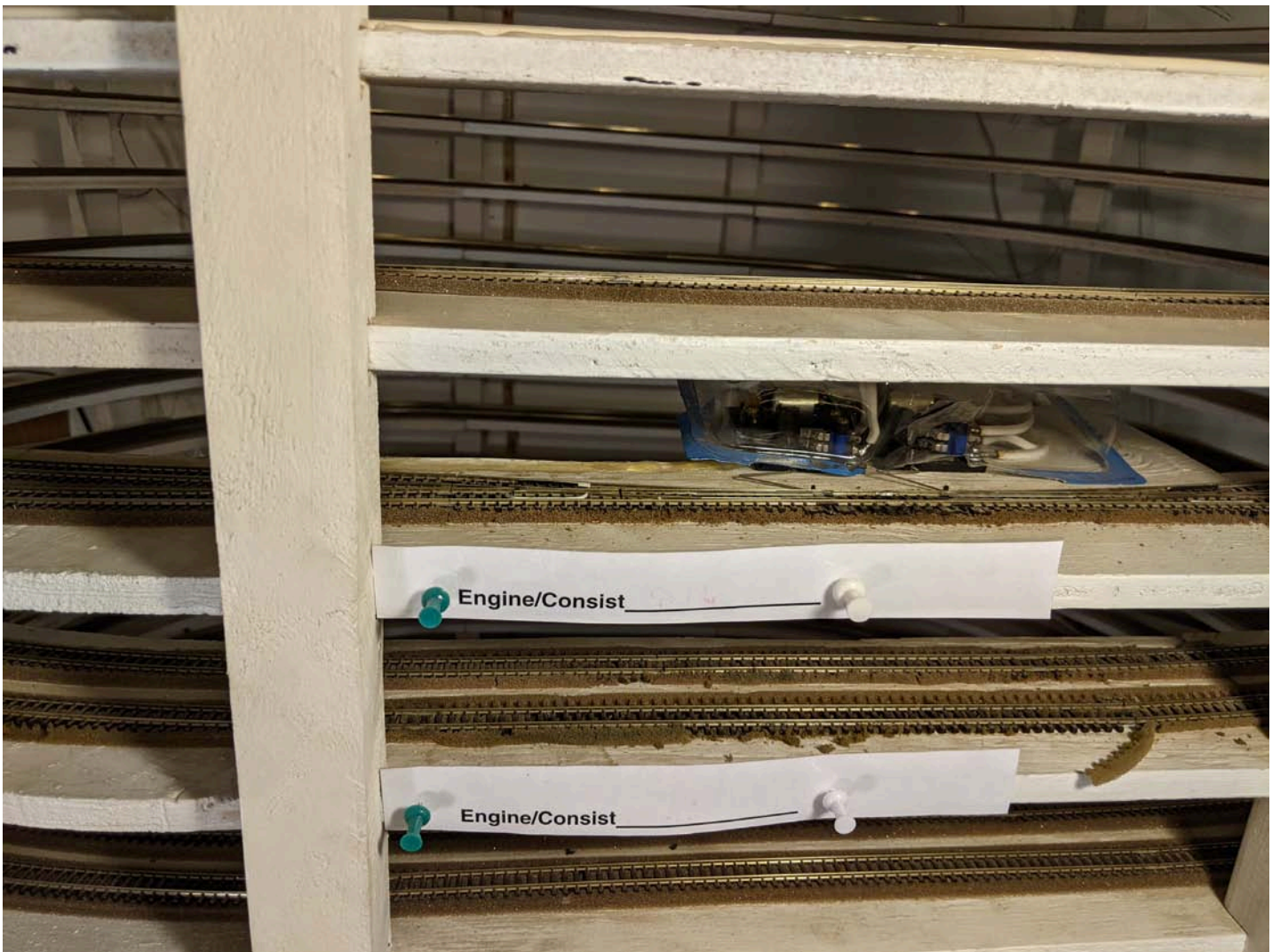
Above. Depending on the task needed to be accomplished, the track varies between single and double tracks, crossovers, etc. After many years about \frac{1}{4} of the Peco foam roadbed has deteriorated. It can easily be replaced.
