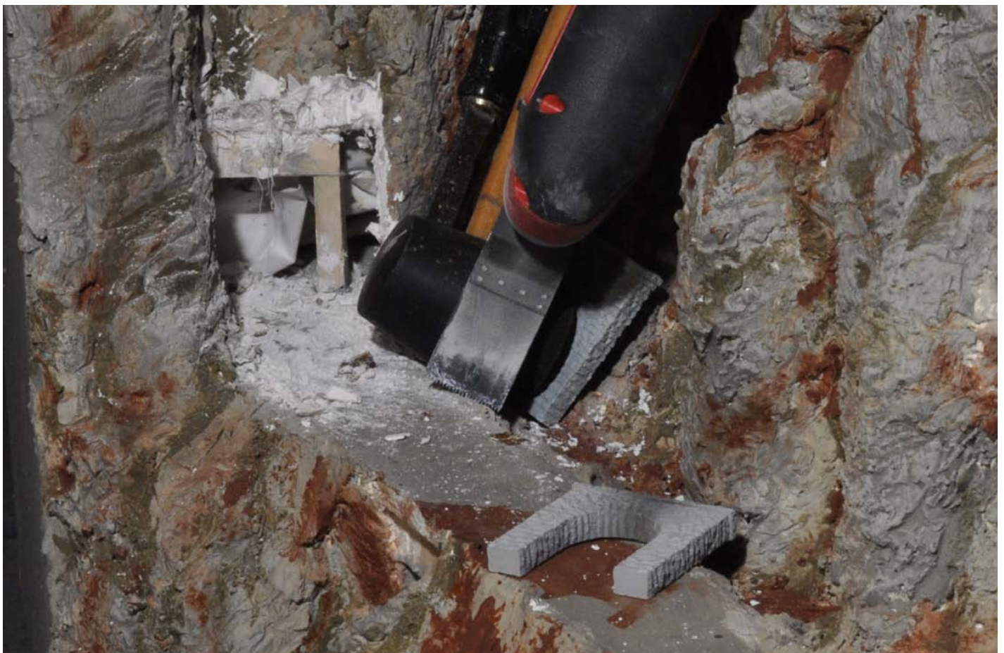
Above. Yea... I had to do more clean up than I originally thought. But this is a lot easier than using a chisel.
