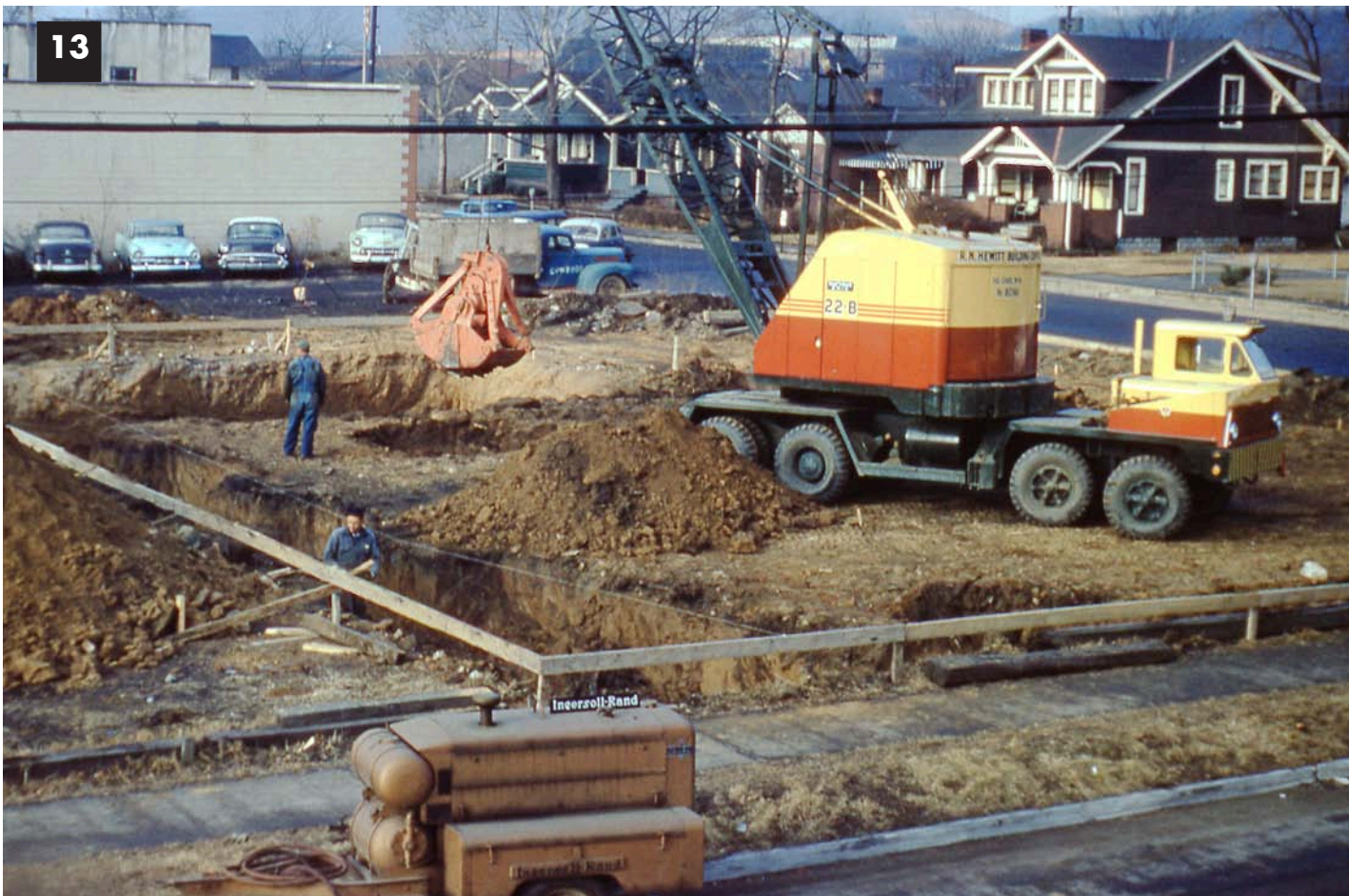
13. This 22B Bucyrus Erie transit crane can be kitbashed using a Langley E31a kit and a #2065 Bantam Excavator Truck from Railway Express Miniatures. Transit cranes were commonly used at excavation sites before hydraulic excavators were available. The color paint scheme of this 22B crane was common throughout all of the Bucyrus-Erie 22b production runs.
