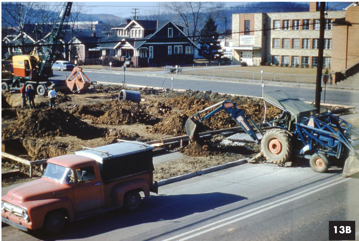
13. This 22B Bucyrus Erie transit crane can be kitbashed using a Langley E31a kit and a #2065 Bantam Excavator Truck from Railway Express Miniatures. Transit cranes were commonly used at excavation sites before hydraulic excavators were available. The color paint scheme of this 22B crane was common throughout all of the Bucyrus-Erie 22b production runs.
