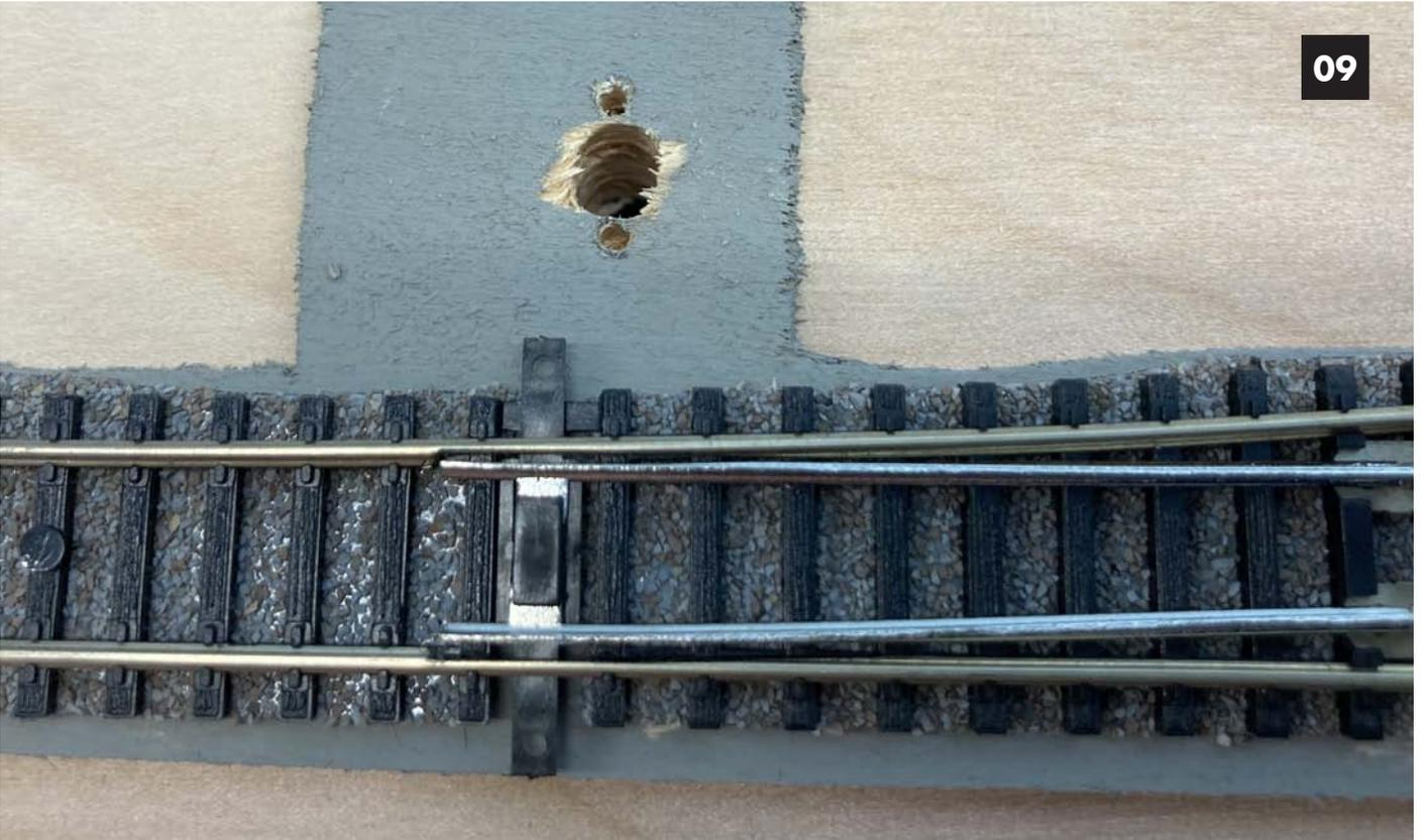
Image 09. Next a larger center hole is drilled. I use a 7/32" drill.
