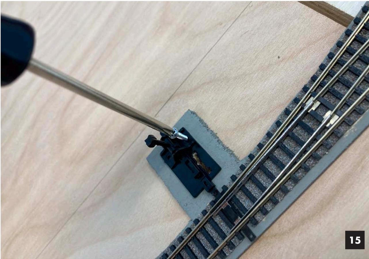
**Image 15.** Carefully install the mounting screws.
