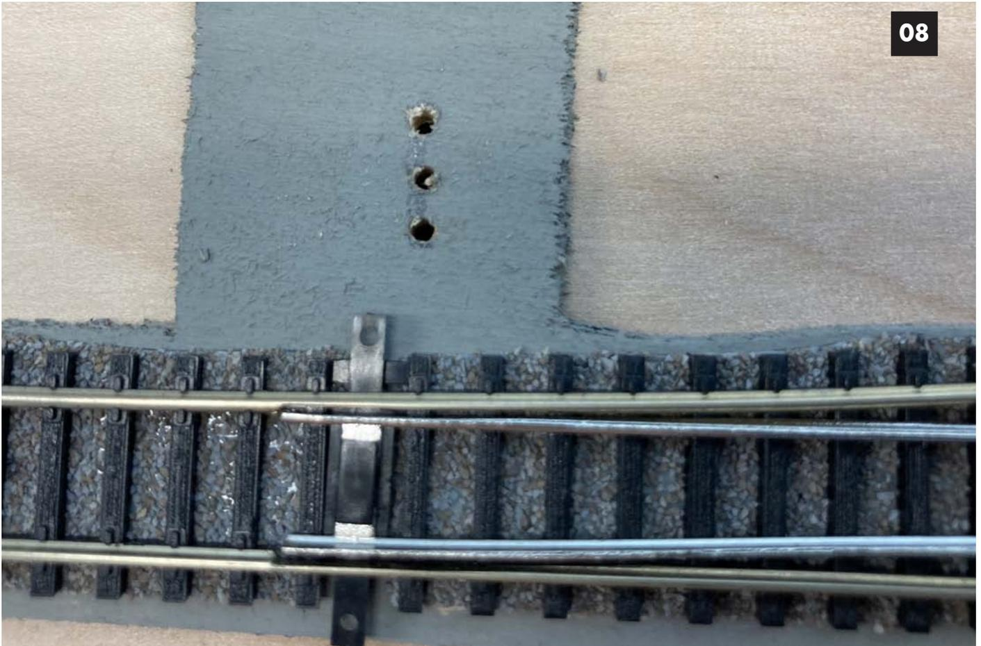
Image 08. Three holes are drilled. I use a #51 drill.
