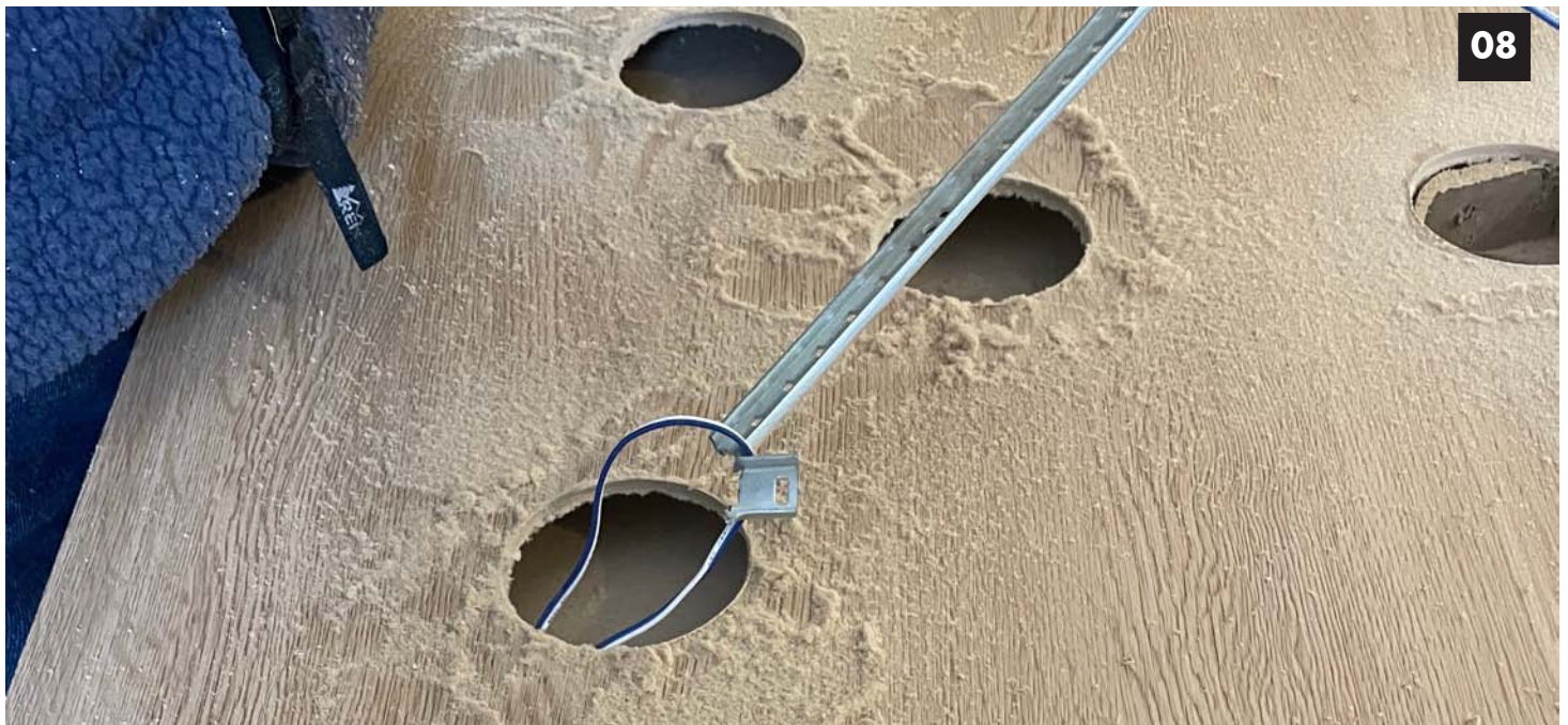
Image 08. Bill improvised a tool to grab and bring wires to the hole on top near the Euro connector.
