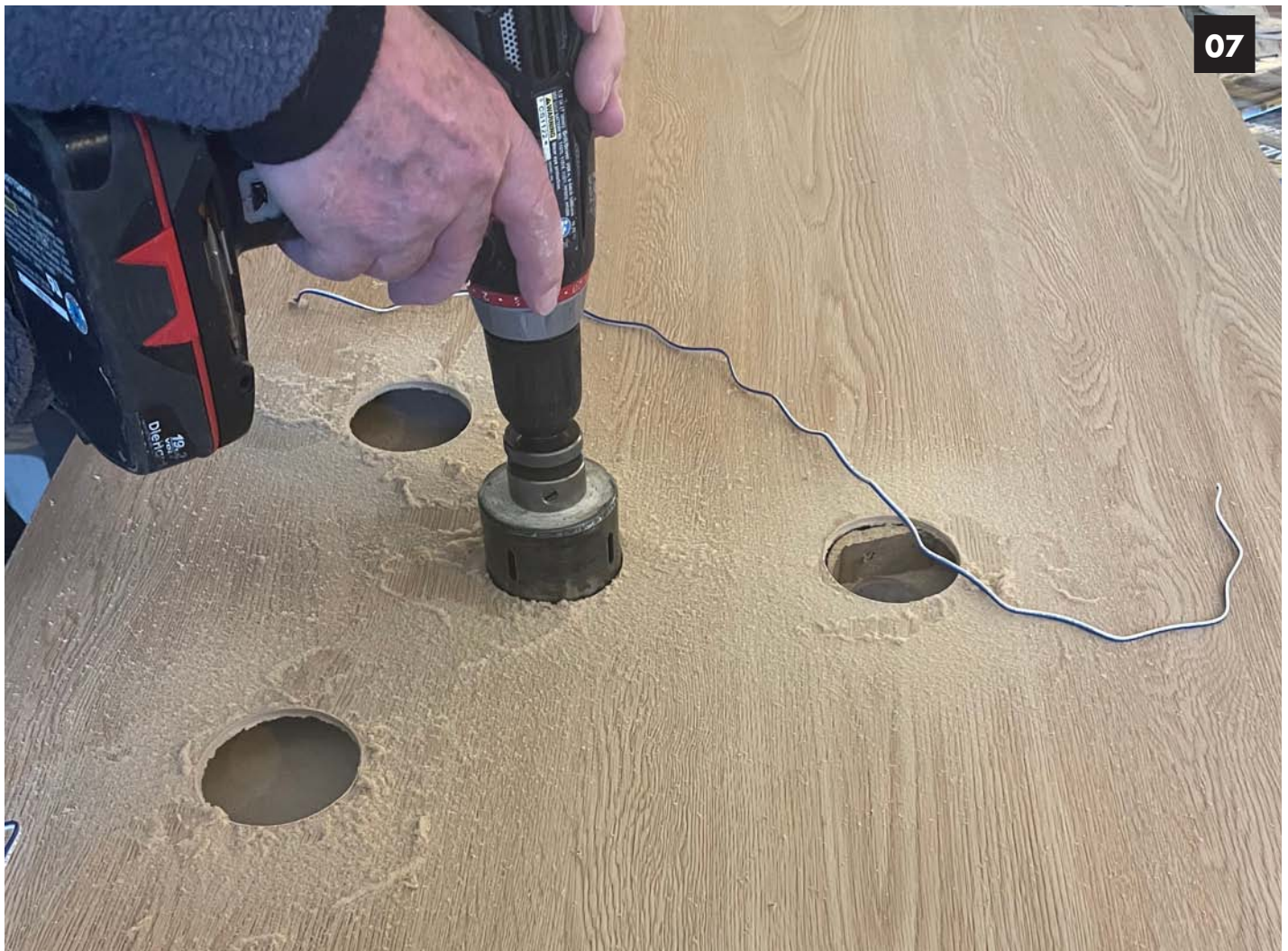
Image 07. This is the bottom of the door. Bill is drilling access holes. The goal is to have all the wires inside the hollow core door. The drill bit is from a set of door bits.
