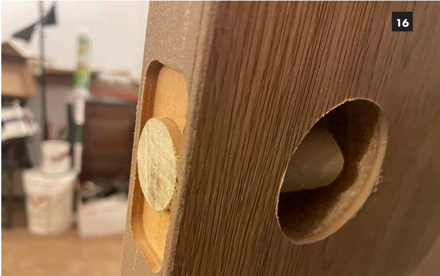
Image 16. Bill started with shaving down a dowel and inserting it into the latch. This also extends into the main hole where the new hole filling pieces will be attached.
