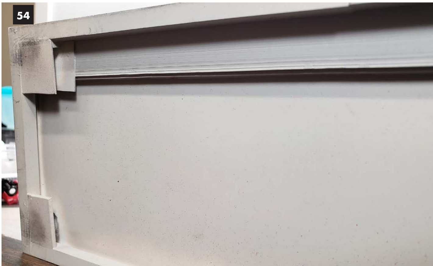
Image 54. Here we see the magnets buried in the foundation. These are to hold the building down to the layout and parking area snug to the dock. An interesting fun fact is something
