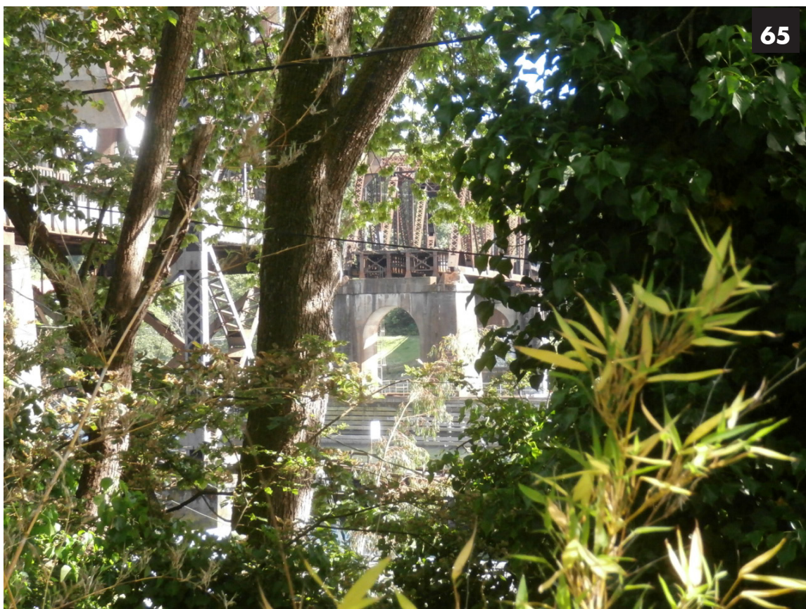
Image 65: View of the concrete piers supporting the south fixed span.
