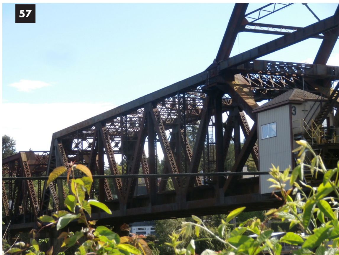
Image 57: The lifting span looking south.
