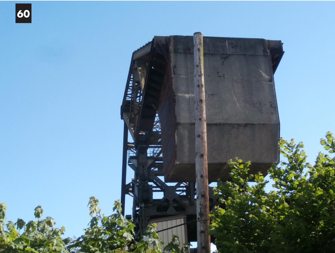
Image 60: View of the counterbalance looking south from Seaview Ave NW.
