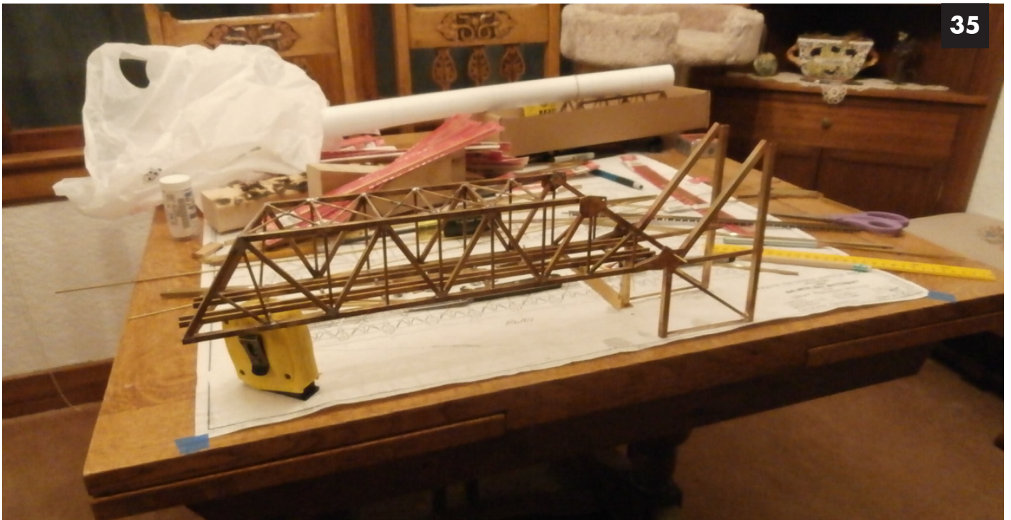
Image 35: Lifting span and north tower together. This step is important to get the right geometry for the trunnion pins and track separation points.
