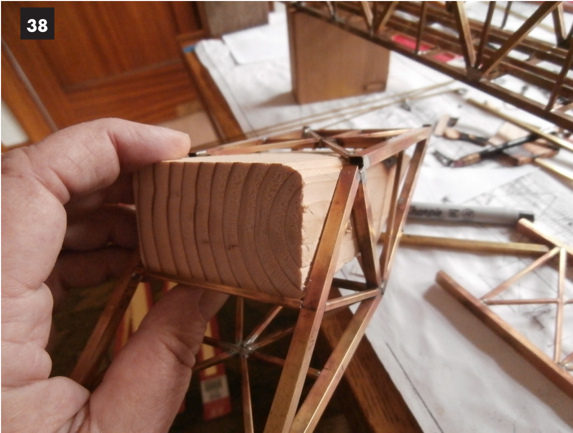
Image 38: The counterweight side frames are secured to a smaller section of 2 x 4 wedge cut to hold the frames at the proper width to operate at the top of the north tower. This attempt ended when the block was built into the completed frame.
