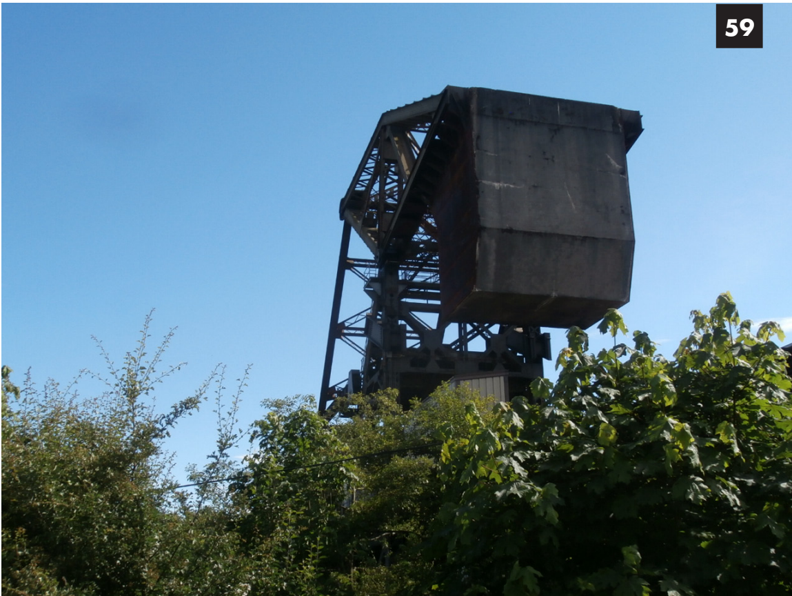
Image 59: The counterweight weighs 1,000,000 pounds to balance the lifting span.
