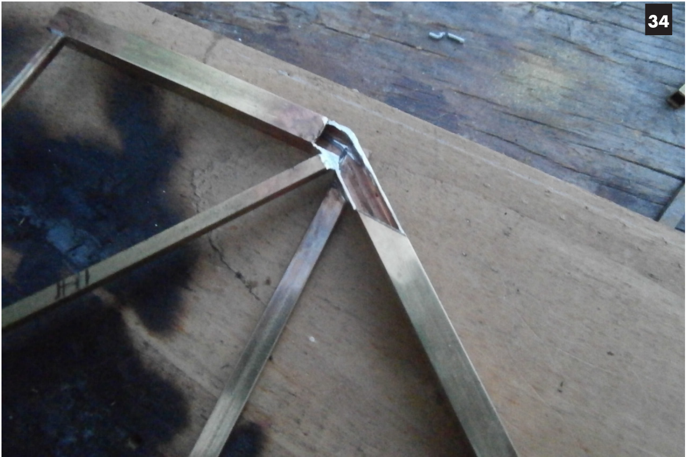
Image 34: Cutouts for the North tower gusset plates.
