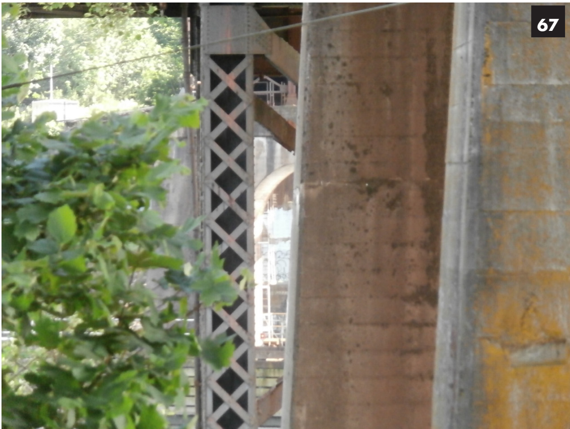
Image 67: Looking south through the trestle
