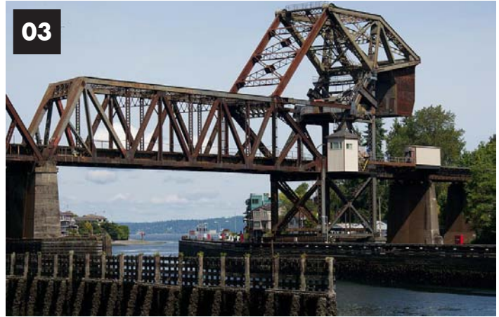
Image 03: Bridge closed looking northwest.
