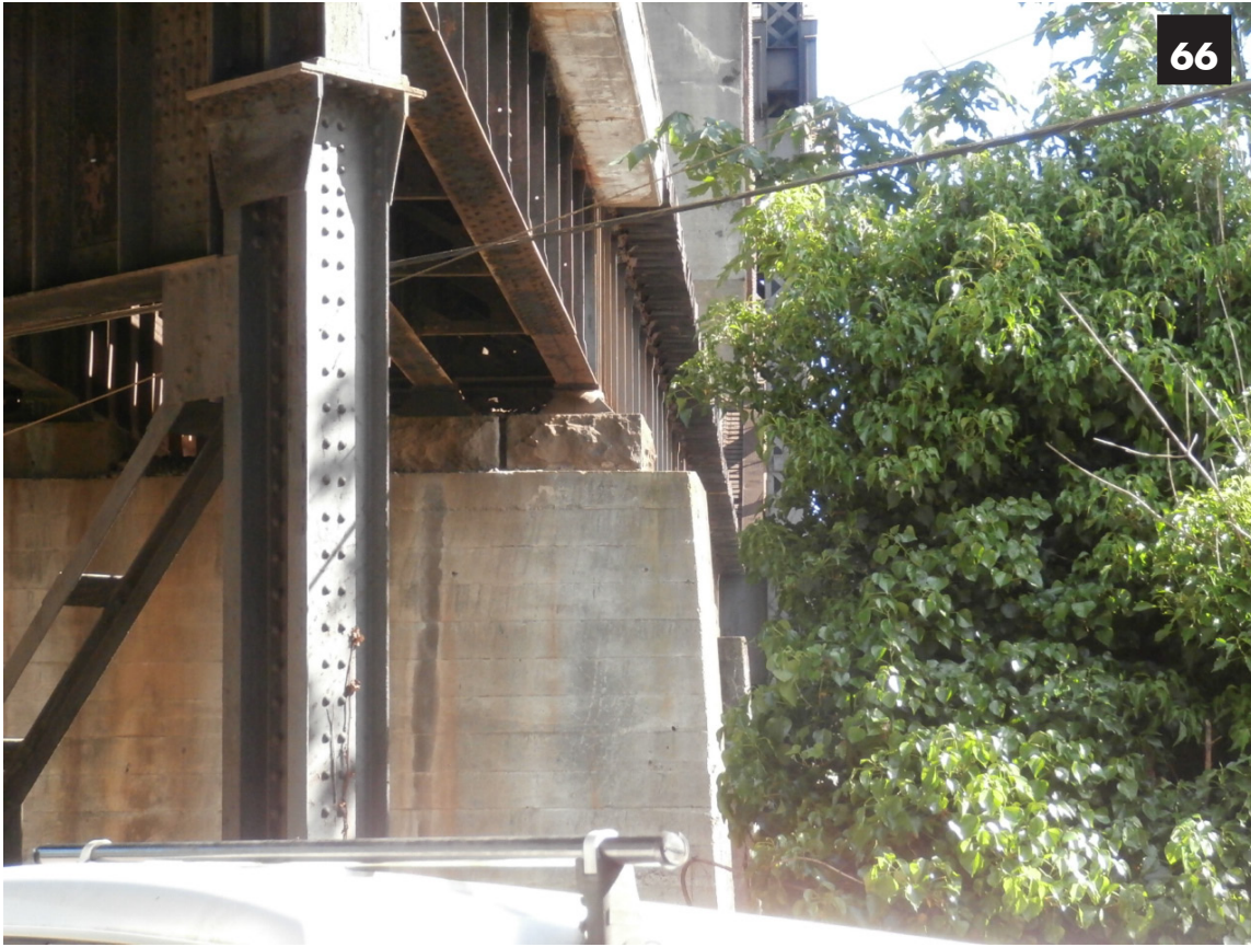
Image 66: Trestle support pier on the north side of the north tower.
