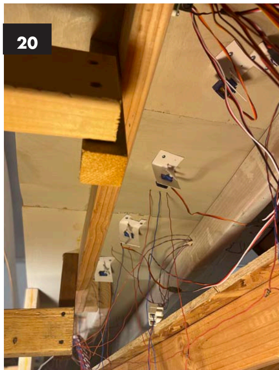
Image 20. The Servo brackets installed under Portland yard.
