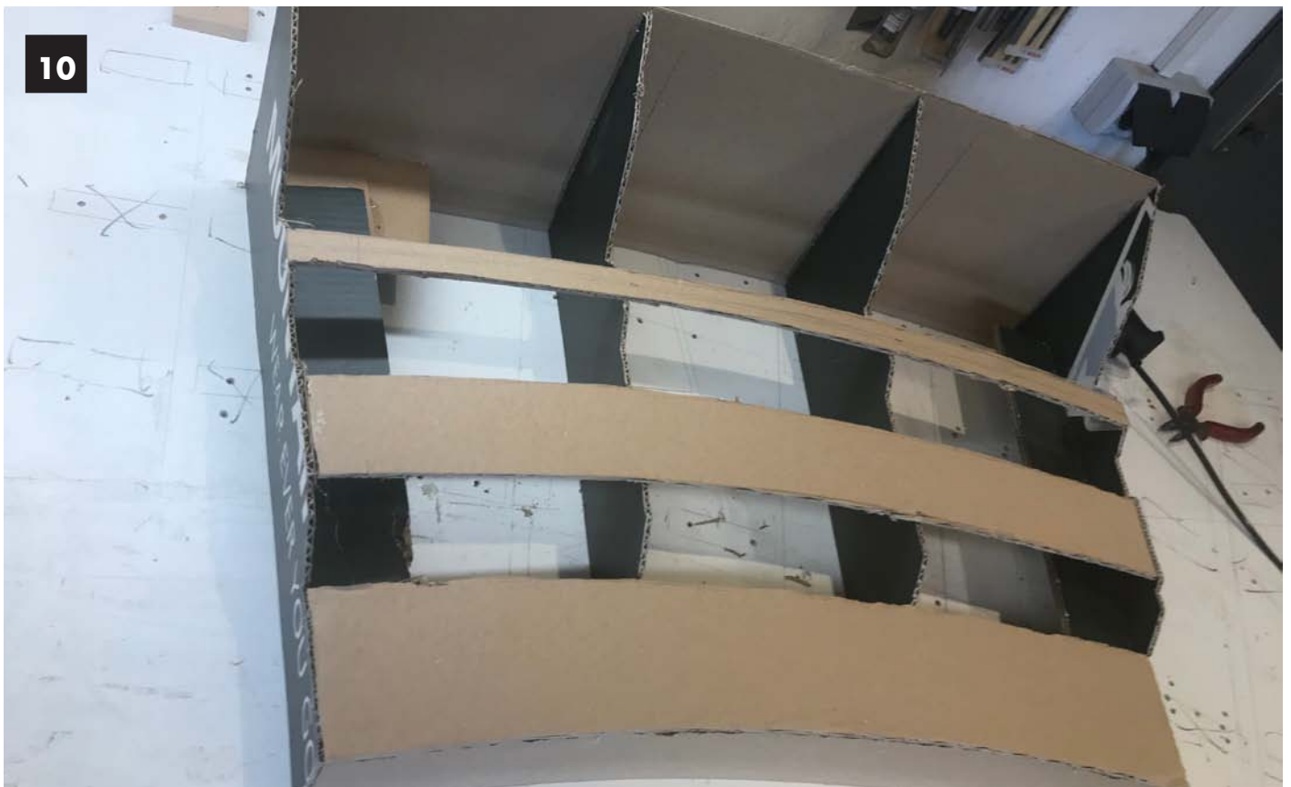
Image 10. Construction followed the same process as for Module 1.0 . Again the hot glue sped up things, though be careful not to get glue on your hands. Wearing gloves is a good precaution against burns.
